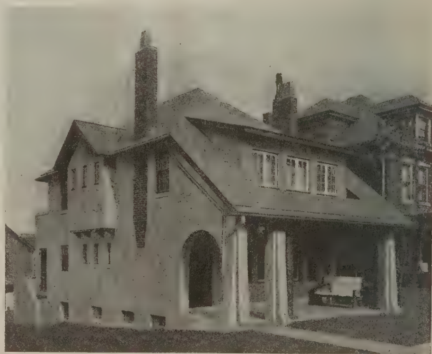
HOUSE OF DR. J. G. B. FITZ-HUGH, McKEESPORT, PA. THOMAS A. RUSSELL, ARCHITECT STUCCO ON STANDARD WALL TILE. WALLS BELOW GRADE ARE OF CONCRETE. THE ROOF IS OF SLATE.
